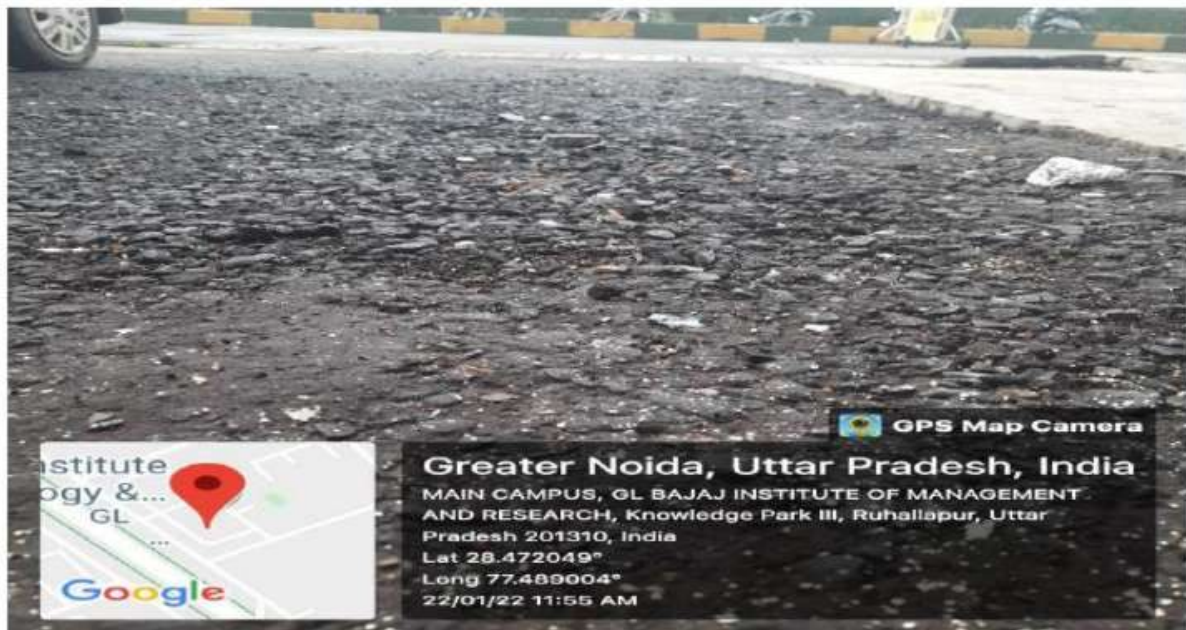
Use of plastic waste as plastic road in campus
